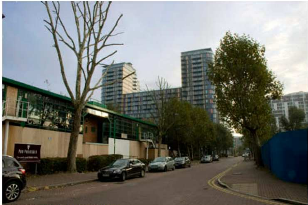
Existing View from North-West of Building
