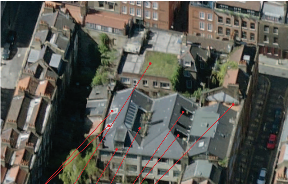
Figure 2: 6-10 Princelet Street viewed from the east
